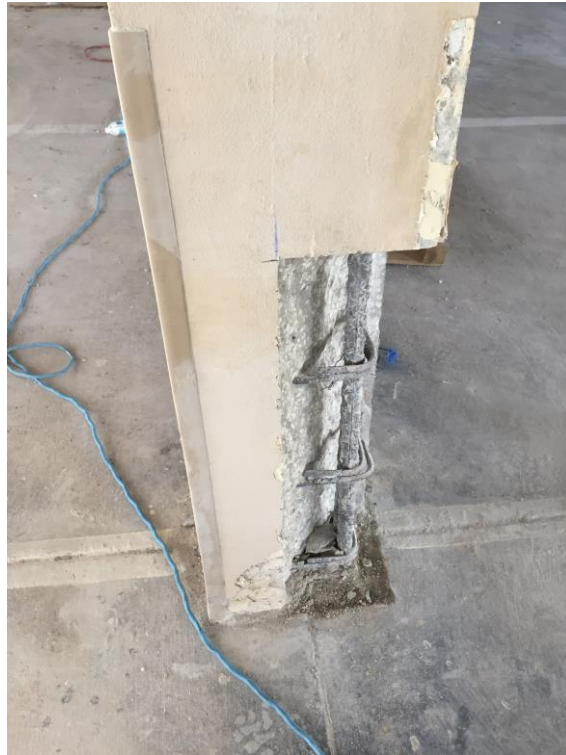
Picture 3: Column excavation
