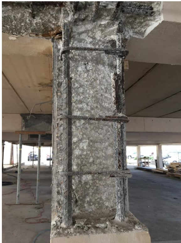
Picture 2: Column excavation
