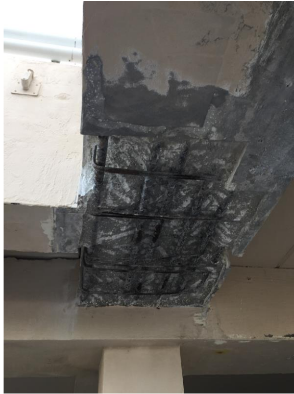
Picture 1: Beam excavation
