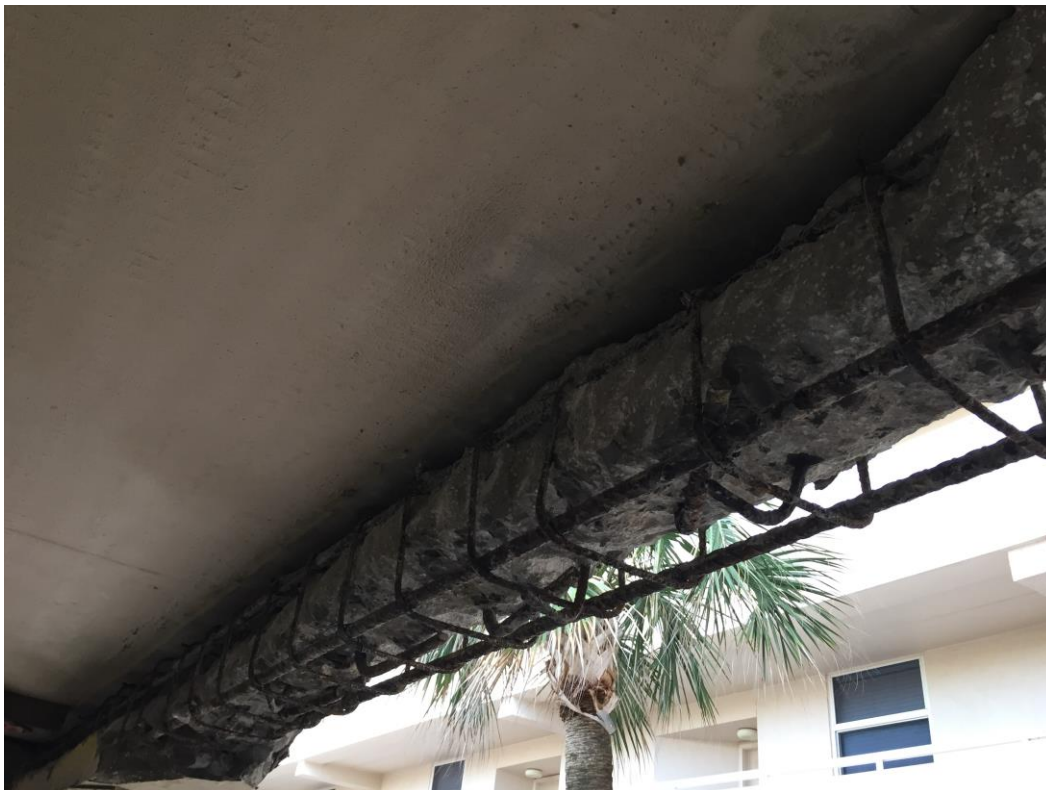
Picture 4: In-progress concrete repair
